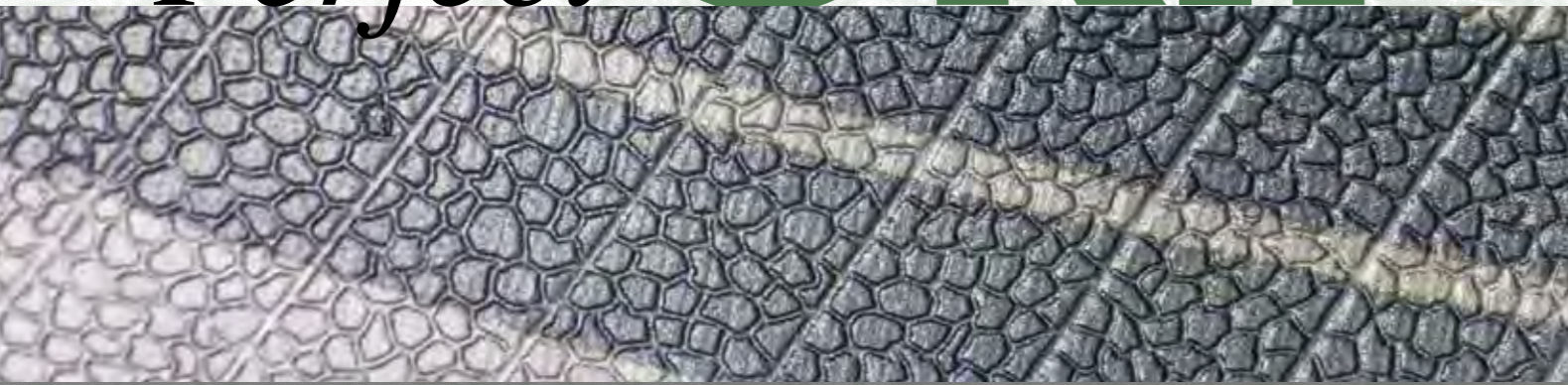
Partially cleaned inner liner
